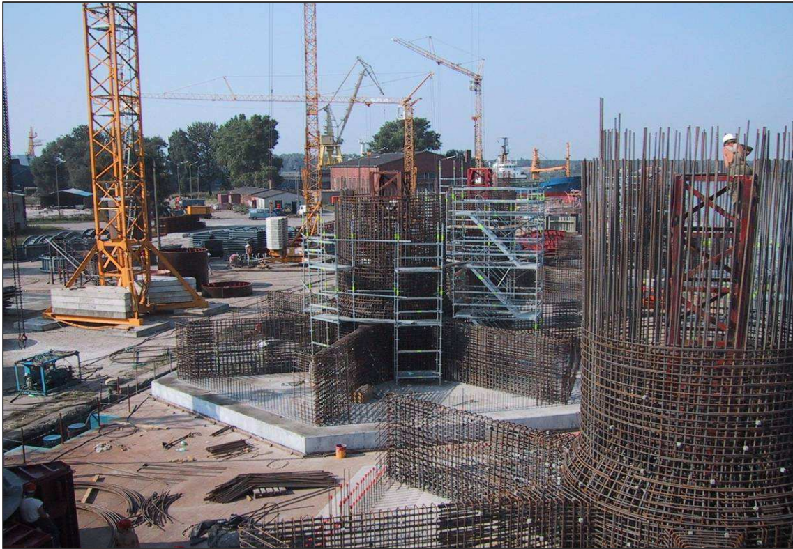
Figure 3. Concrete gravity offshore foundations during construction.
