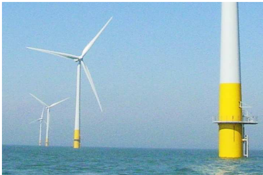
Figure 1. The support structures for the wind turbines at Kentish Flats are designed and certified to DNV-OS-J101
